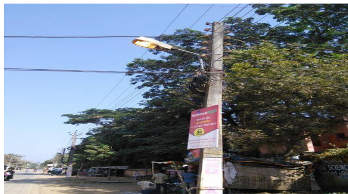
Picture of Indian street light which is 'ON' in afternoon Picture Credits: Amul Jalan.
